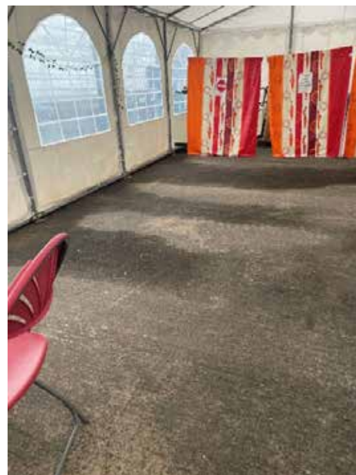
Evidence of water build up on the concrete floor the marquee sits on
