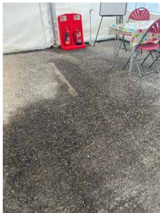
Evidence of water build up on the concrete floor the marquee sits on
